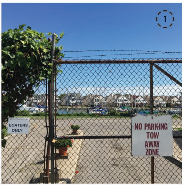
GRAYHAVEN MOORING FACILITY FENCE
