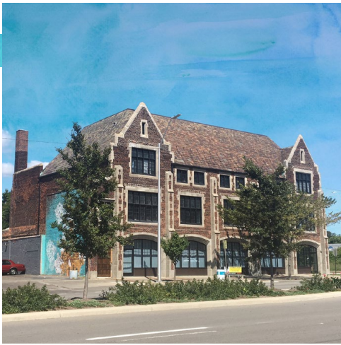
Figure 17: St. Columba Parish Building
