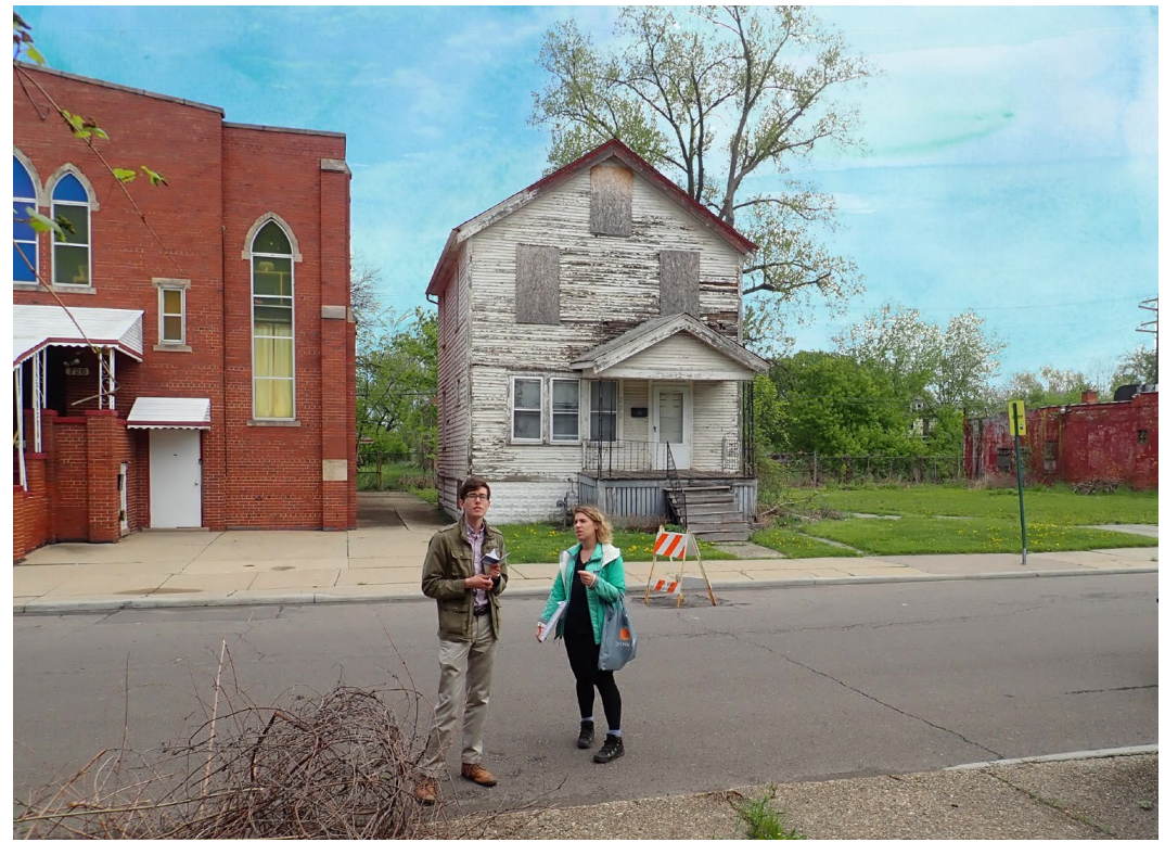
Figure 10: On the job in Jefferson Chalmers
