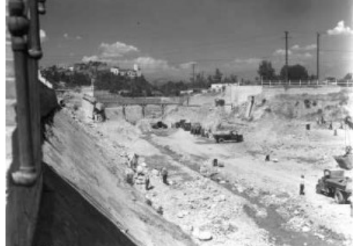
Davison Freeway Construction Detroit 1941
