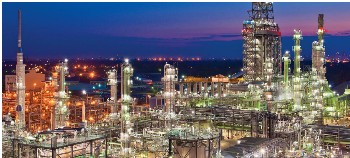
Figure 153: Marathon Petroleum 12800 Toronto Street, Detroit
