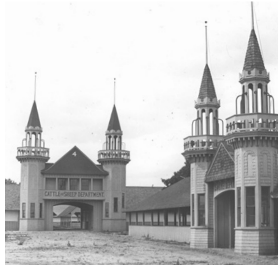
Figure 25: A portion of the architecture of the exposition
