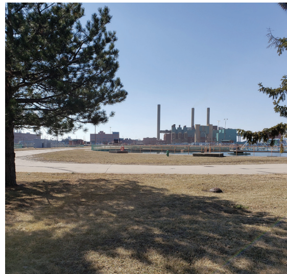
Figure 124: Wastewater Treatment Plant 9300 W. Jefferson
