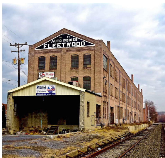
Figure 73: The Fleetwood plant shortly before its demolition
