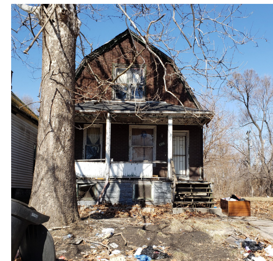
Figure 96: Marquez Residence 8334 Vanderbilt St
