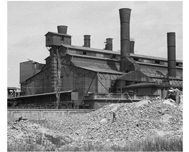
Figure 165: Powiśle Power plant before renovation
