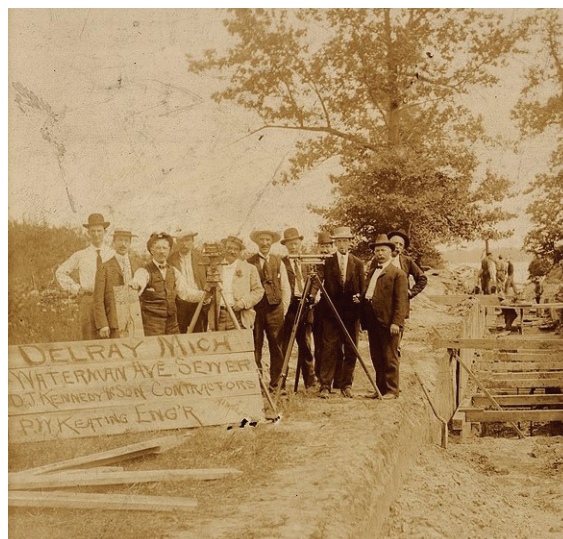
Figure 94: Construction of the Waterman Ave. sewer
