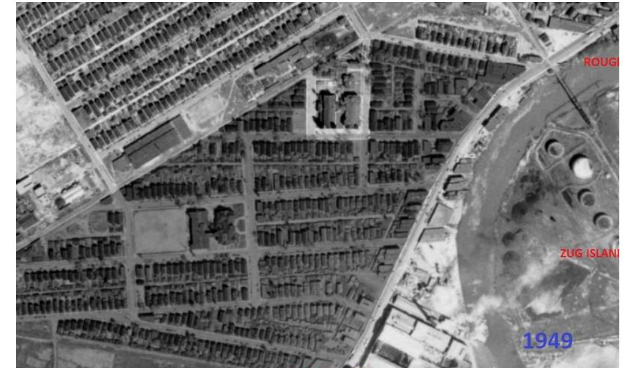
Figure 64: Shaded area was demolished for the Detroit Wastewater Treatment Plant
