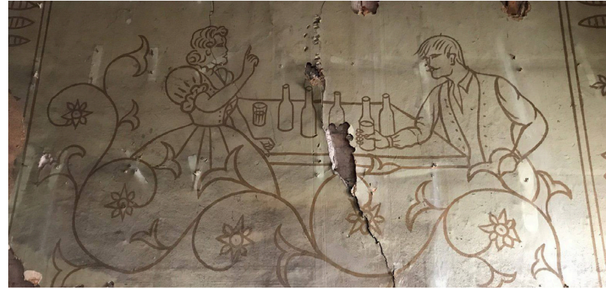
Figure 63: The original walls of Kovacs Bar discovered during the demolition
