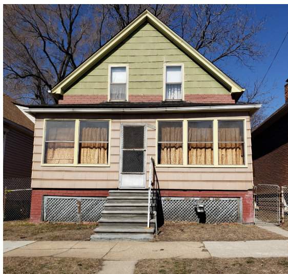
Figure 101: Vinczler Residence 8056 South St
