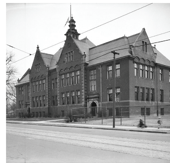
Figure 95: Gillis Elementary School on Junction
