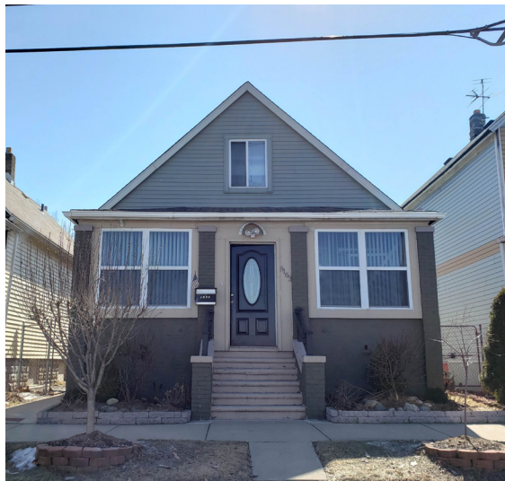
Figure 107: Orozco Residence 8163 Melville St
