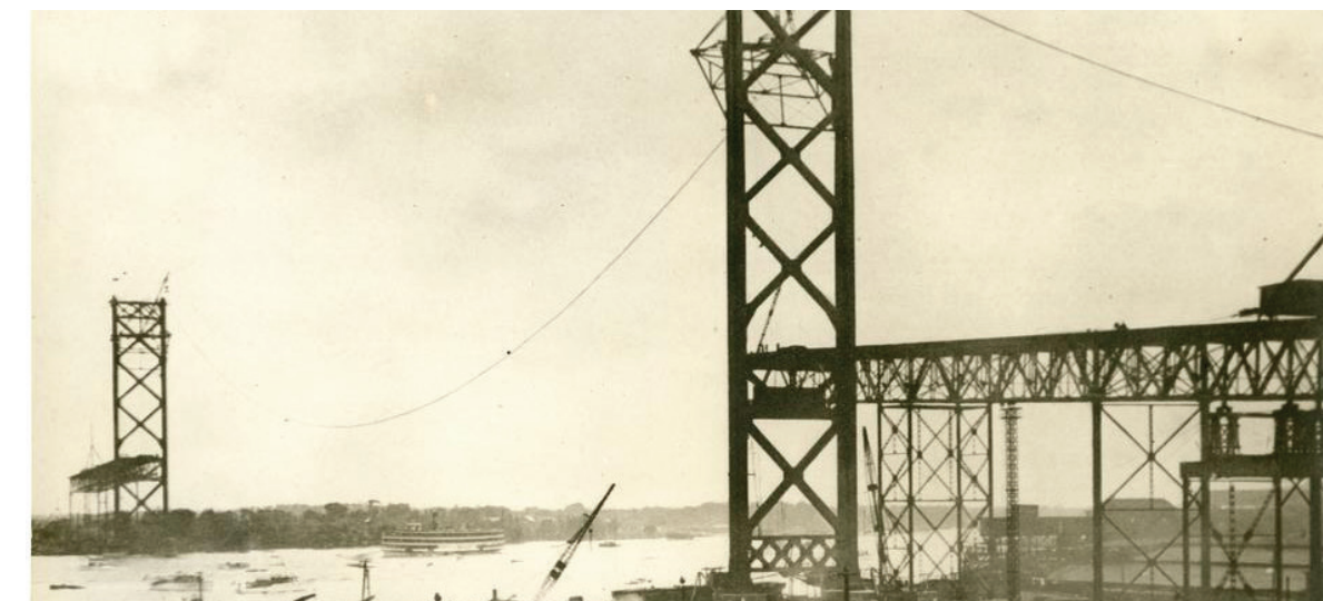
Figure 97: Construction of the Ambassador Bridge
