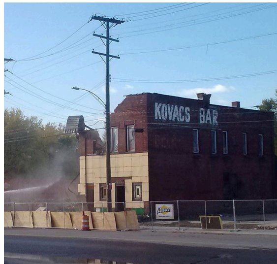
Figure 132: Kovacs Bar demolition
