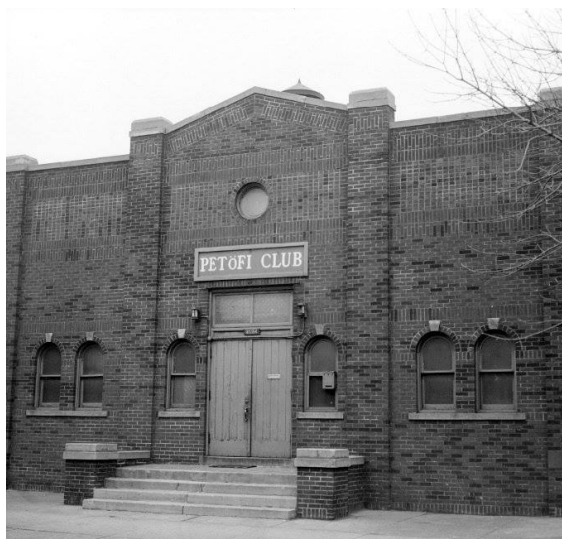
Figure 91: Exterior of the Petofi Club 1952
