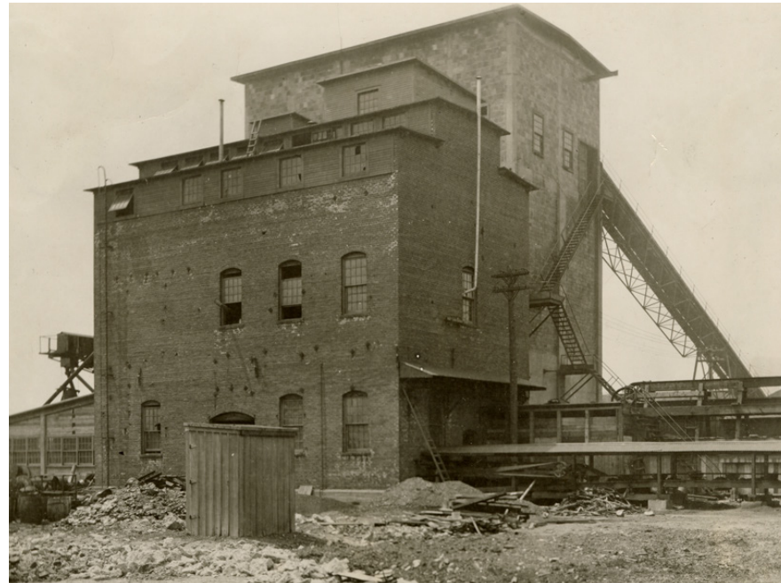
Figure 38: Briquetting plant and coke bins
