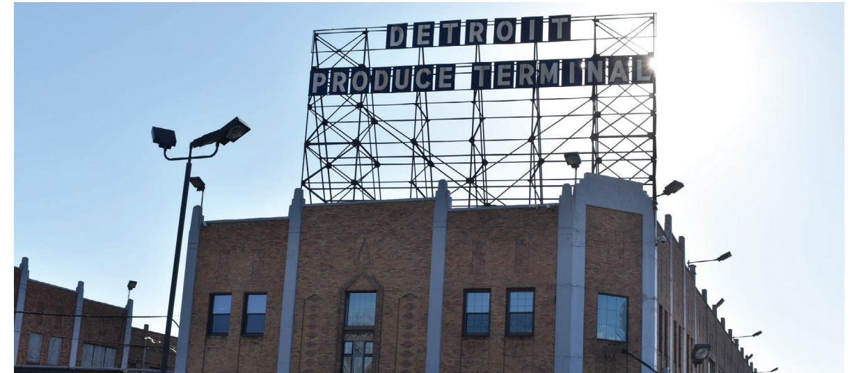
Figure 142: Detroit Produce Terminal 7201 W. Fort
