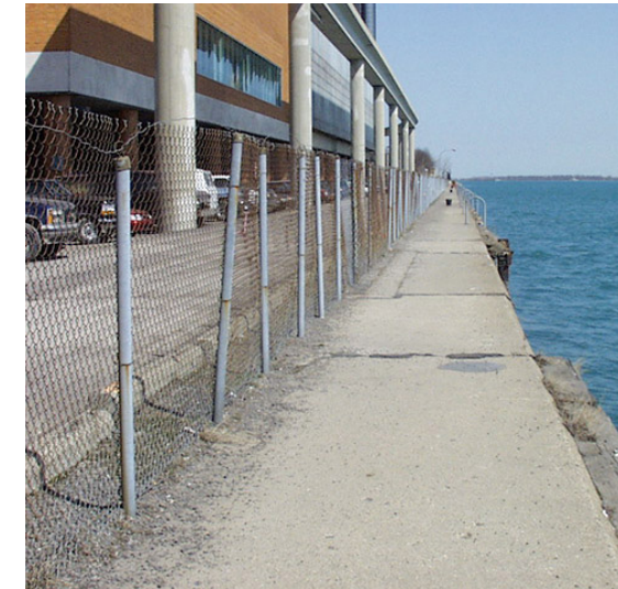
Figure 169: Detroit's Civic Center before renovation
