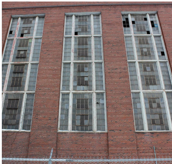
Figure 130: DTE Waterman Substation 708 S. Waterman
