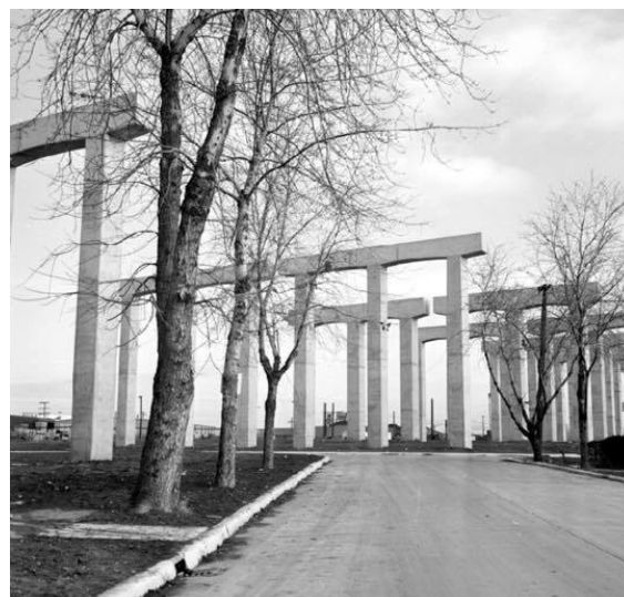
Figure 71: I-75 being built through peoples yards
