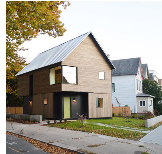
Figure 158: Exterior front of the 2019 Jim Vlock Studio
