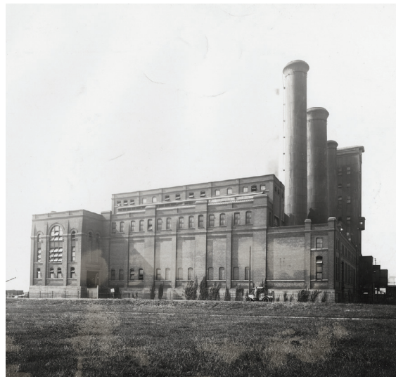
Figure 132: DTE Waterman Substation in 1909
