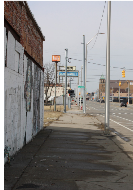
Fig. 1.02 Sidewalk condition along Grand River Ave.
