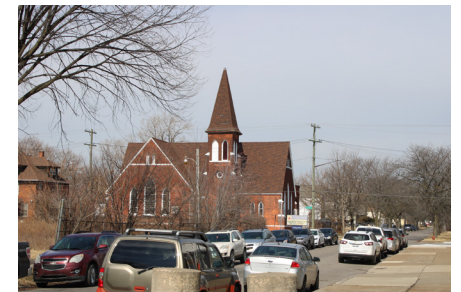
Fig. 5.08 Greater St. James F.B.H. Church located on 18th St.
