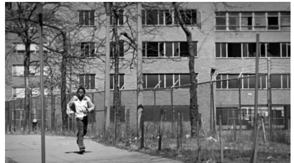
Fig. 2.11 Broken windows and barbed wire fences dot the Pruitt-Igoe project.
