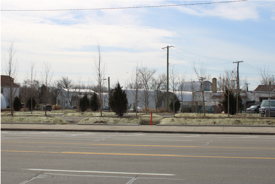
Fig. 5.15 The True North (2017) live-work development designed by Prince Concepts located on Grand River Ave.
