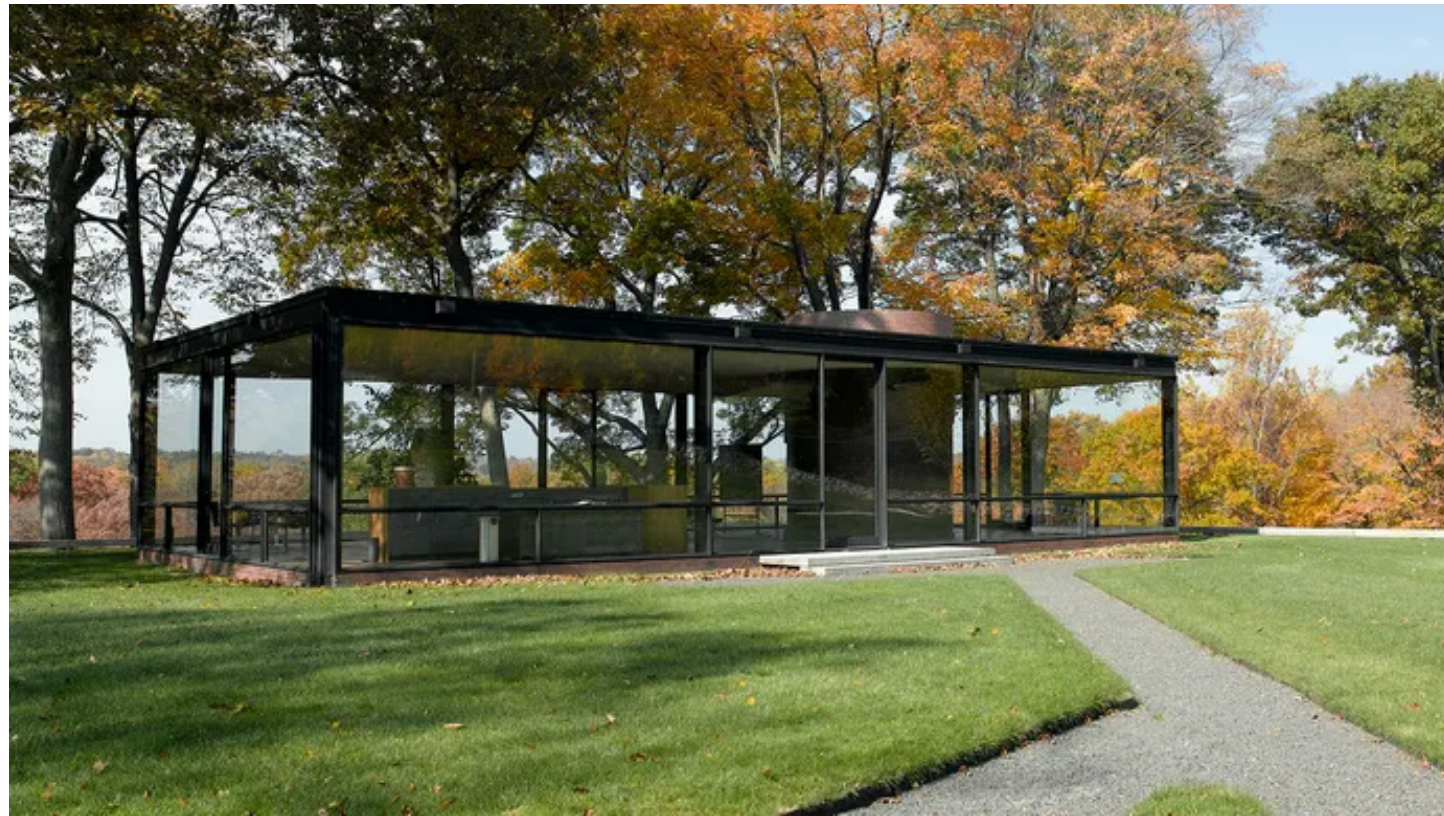
Fig. 2.03 The Glass House (1948-1949) by Philip Johnson
