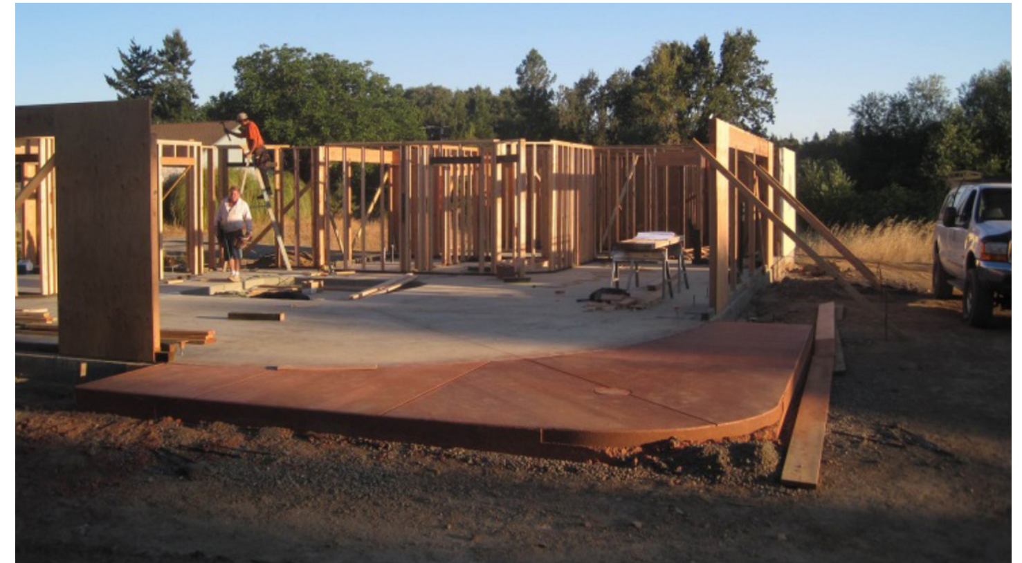
Fig. 7.08 Pomo typology construction process
