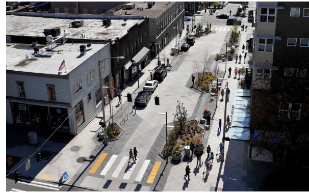
Fig. 5.3.2 – Bell Street AFTER
