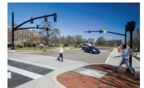
Fig. 5.4.5 – New crosswalks and streetlights
