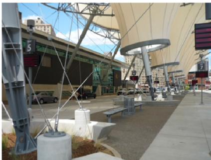
Figure 35. Rosa Parks Transit Center. Source: Innovative Surface Works
