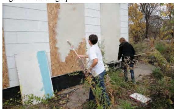
Fig. 28. Application of the base coat of paint
