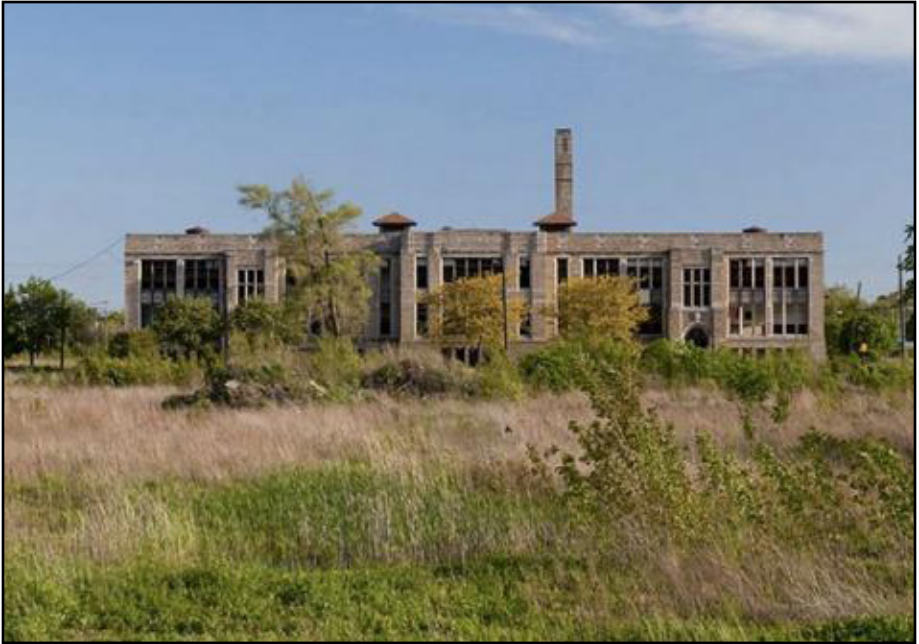
Figure 32: Vacant former Detroit Public School building Source: Loveland Technologies
