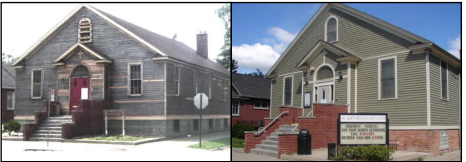
Figures 16 & 17: The All Saints Center before and after renovation Source: Urban Neighborhood Initiatives website
