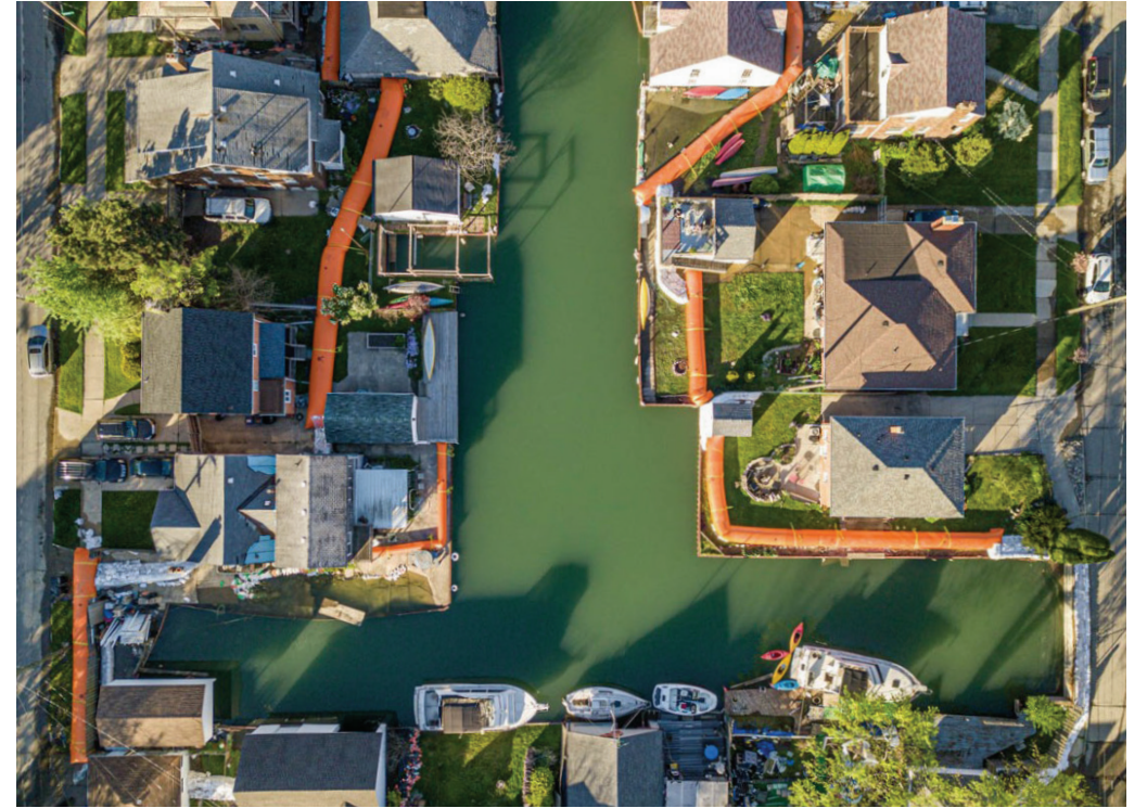
FIGURE 104. Aerial view of "Tiger Dam" flood water mitigation project in Jefferson Chalmers neighborhood in east Detroit (Brian Allnutt)
