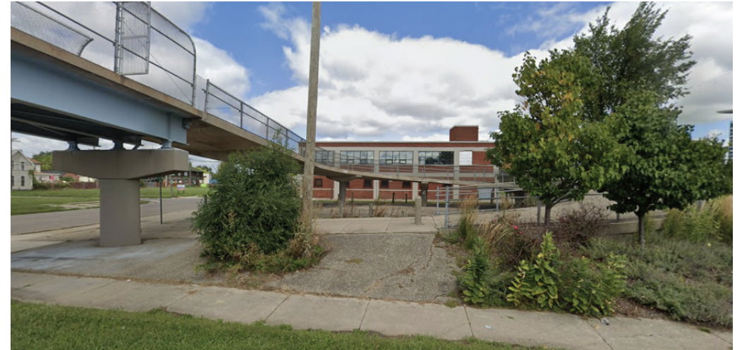
FIGURE 047. Cochrane Street Pedestrian Bridge (Google Street View)
