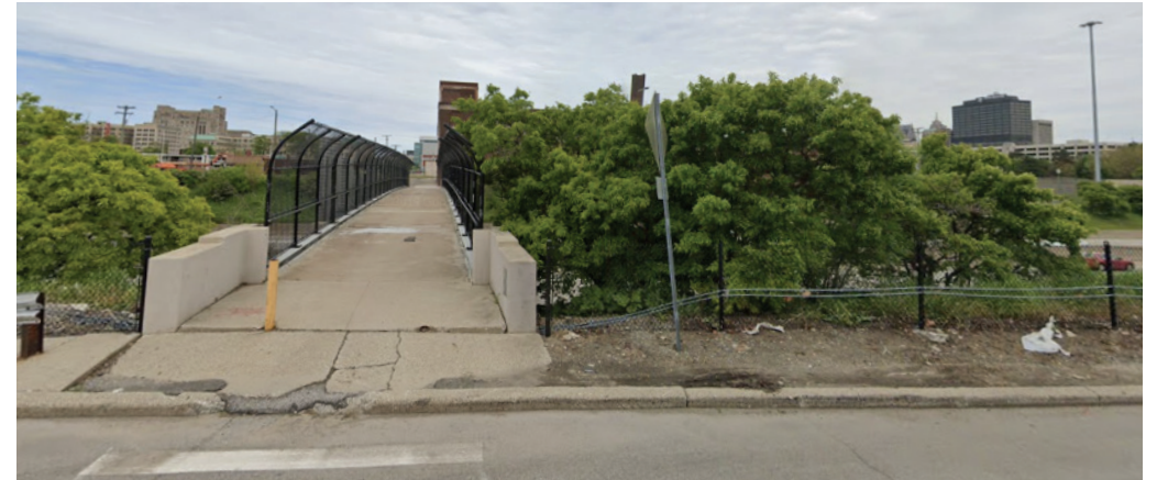
FIGURE 048. Cochrane Street Pedestrian Bridge (Google Street View)
