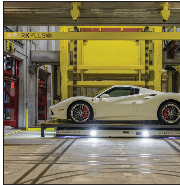
Figure 5.2 - ParkPlus Automated Parking System, LA; Source: ParkPlus
