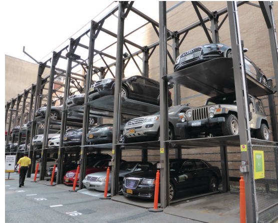
'Saving Space' - Multi-level mechanical stacked parking
