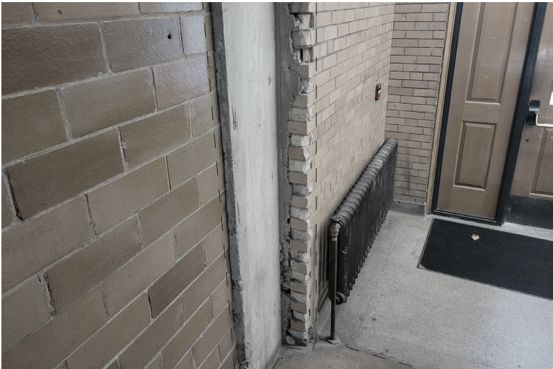
Figure 3.8: A Trace in the Northern Stairwell
