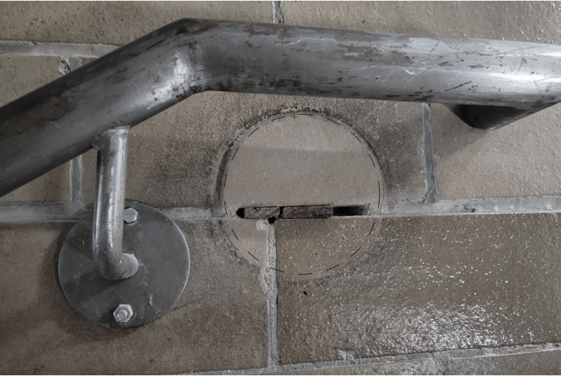
Figure 3.10: A Trace in the Southern Stairwell
