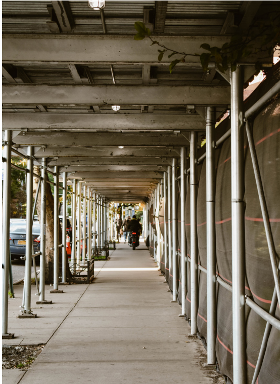
Figure B.17: Scaffolding in Manhattan
