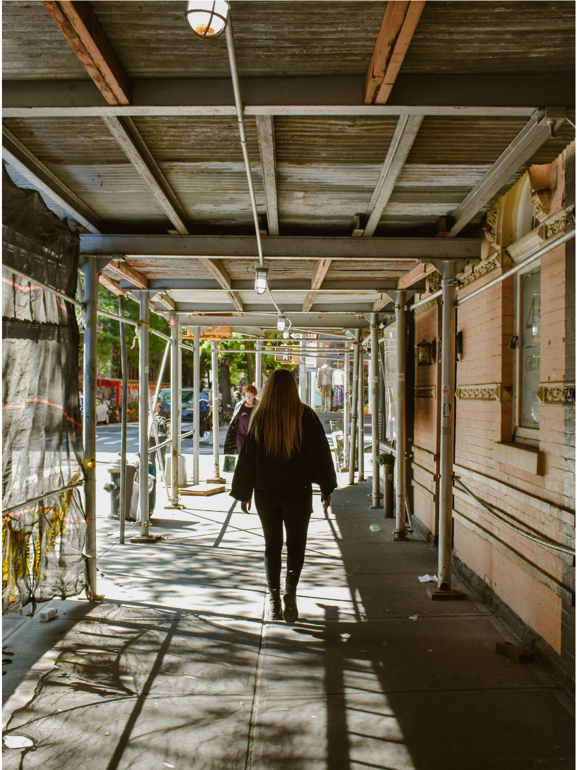
Figure B.16: Scaffolding in Manhattan
