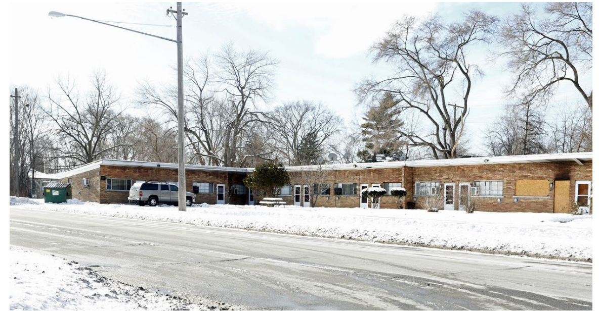
Figure 3.3: View of Deeply affordable housing near 7 Mile/Mound
