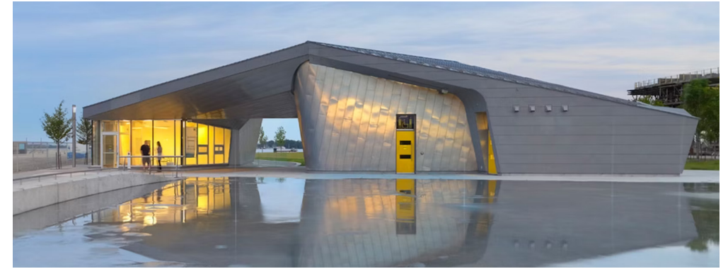
Fig. 2.7, Sherbourne Common Pavilion, Source: Architizer
