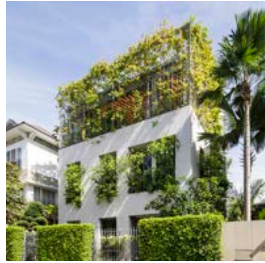
figure 3.3. Stepping Park House.
