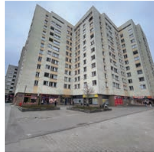
figure 11.6. želazna street - photo 6.
