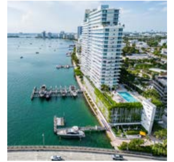
figure 3.4. Bentley Bay - Parking Garage.
