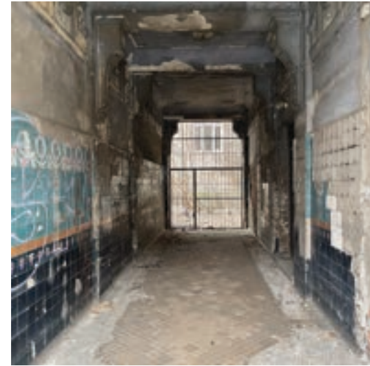
figure 11.5. želazna street - photo 5.
