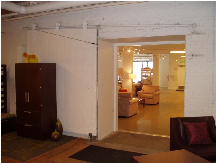
metal fire doors are still required, but are no longer red
