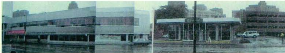
Woodward Ave. across from the site
