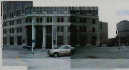
view of office building looking west from Gaslight Restaurant toward Lodge Freeway
