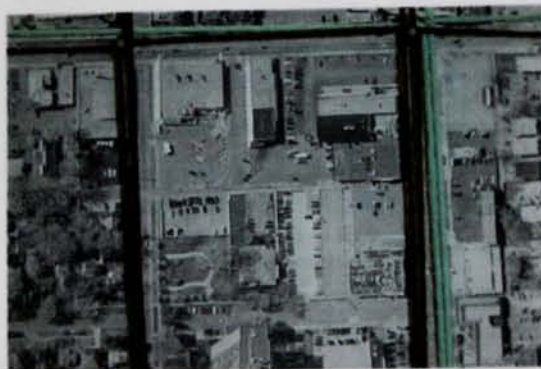
Circulation before Main North Loft Completion
