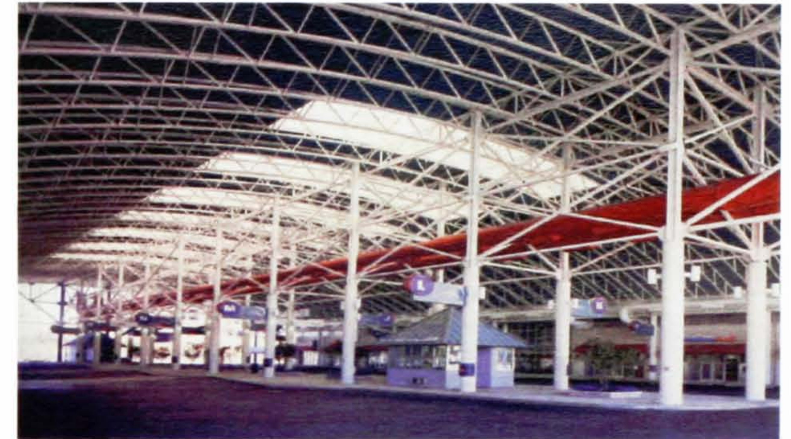
Top: Interior perspective of the bus hub in the Transportation Center. Middle: Exterior view to the bus hub with adjacent program conditions of the city. Bottom: Floor plan of the bus hub depicting the possible movement of the transportation system into the surround context of Charlotte.
