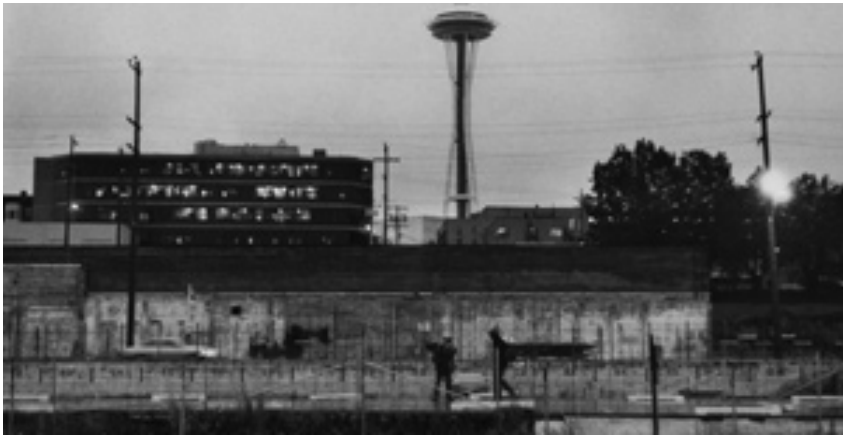
Petroleum Transfer and Distribution Facility (1975)
