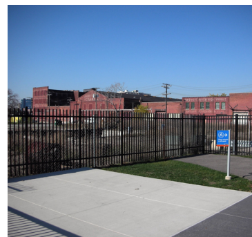
Partially Completed Section of Riverwalk near Parke-Davis
