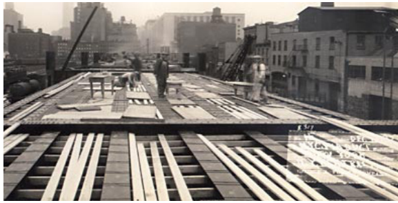
Construction of the High Line - 1929
