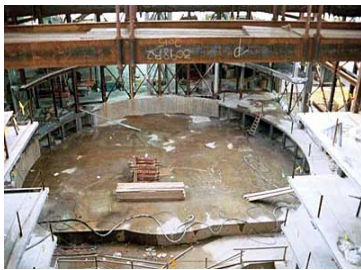
Construction of the radius for the Perelman Theater's revolving stage.
