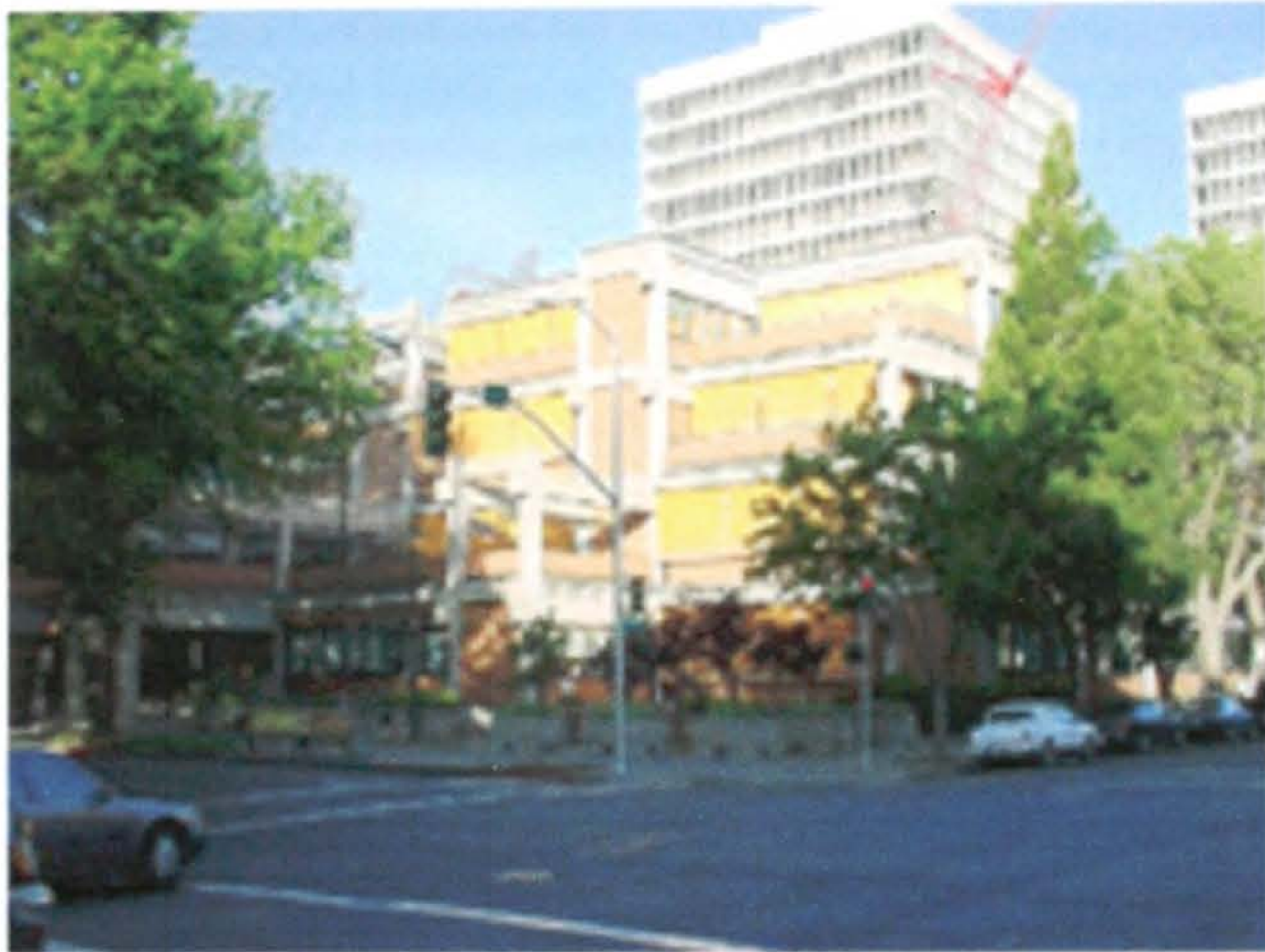
The brightly colored external shades provide protection without creating a formidable appearance
