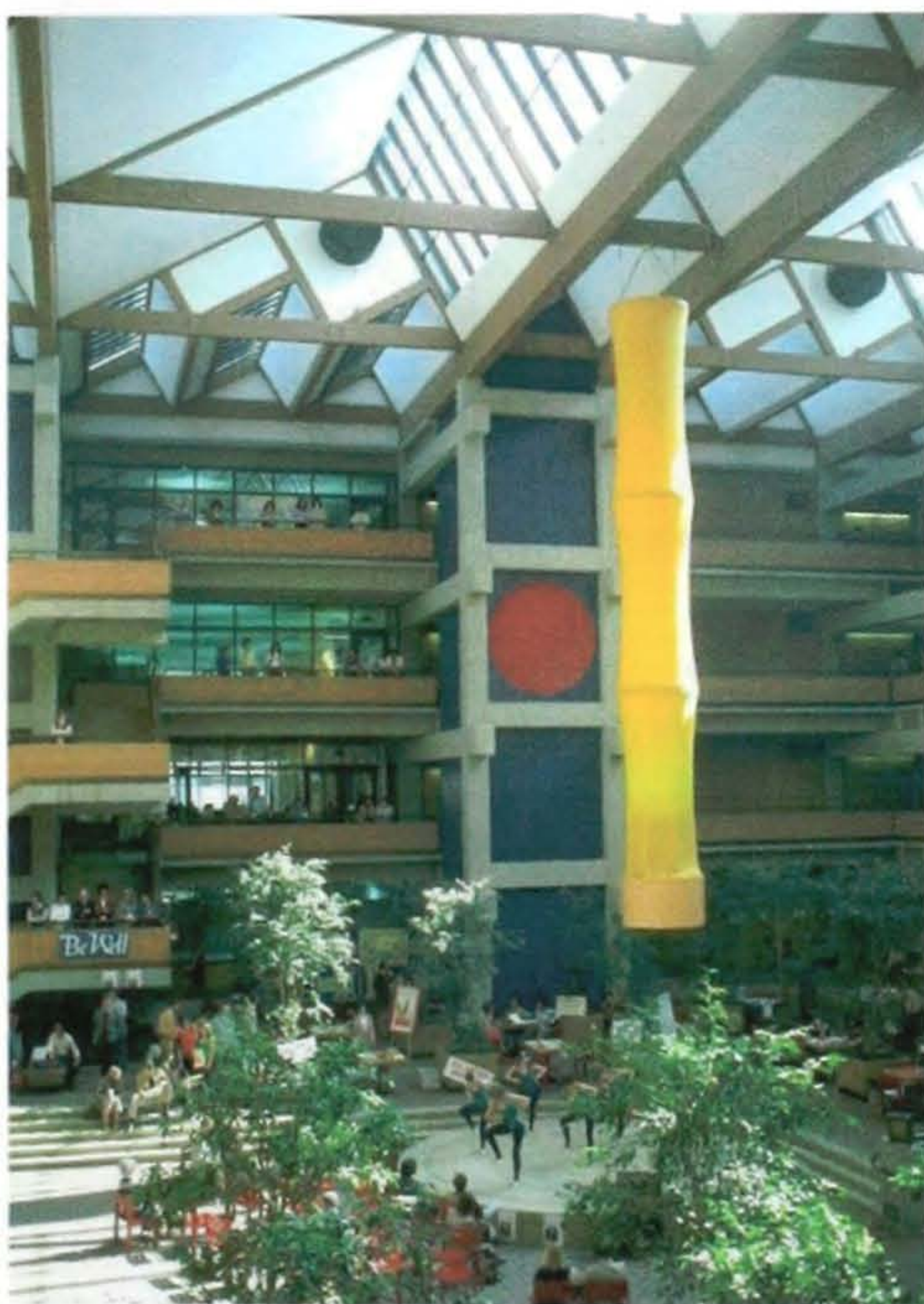
The light and plant filled atrium is the social center of the building as well as a reservoir for coolnight air which circulates through the building keeping temperatures pleasant even on the hottest summer days.
