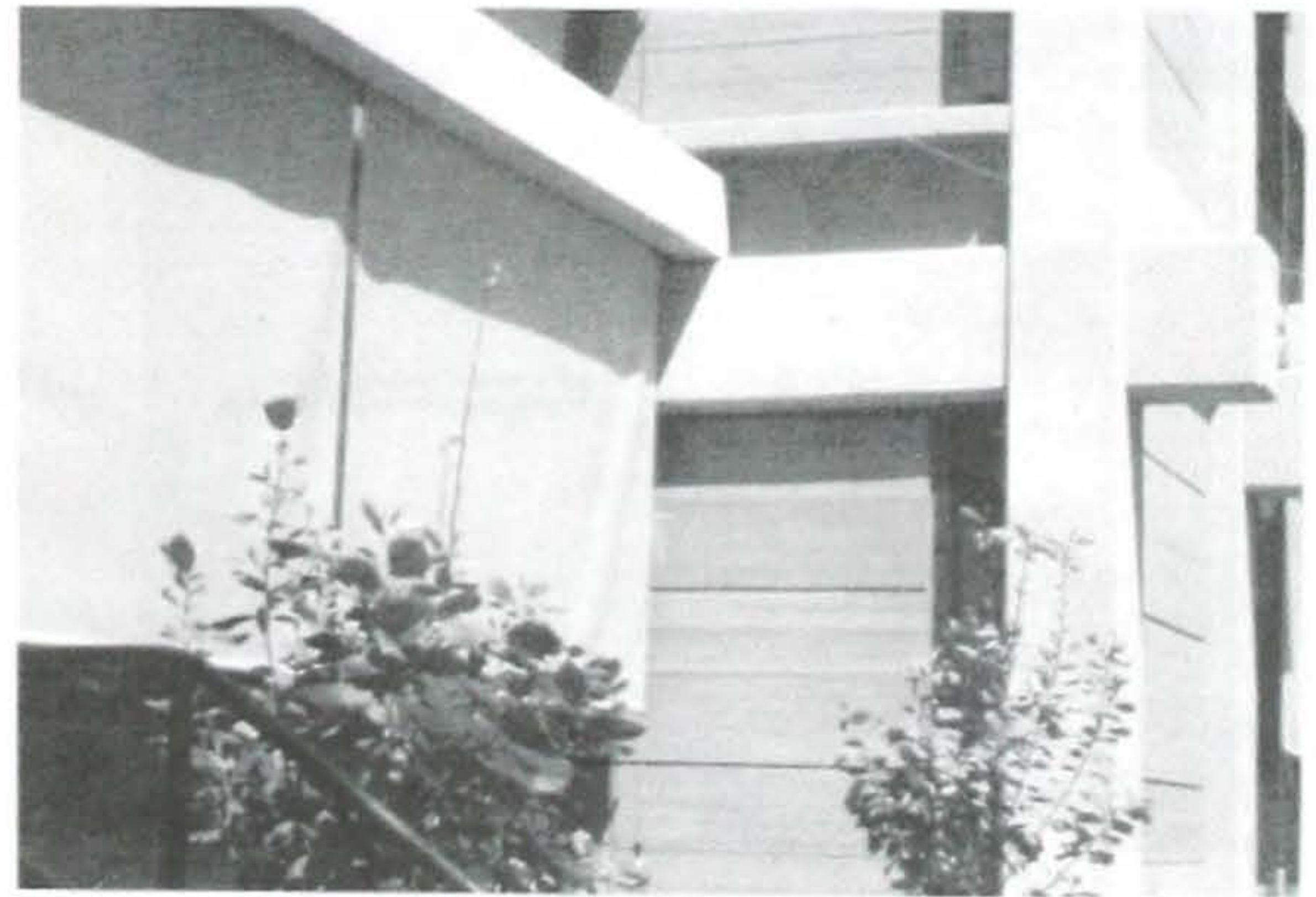
The automated fabric roller shades for the east and west windows are placed on the exterior to minimize solar heat gains
