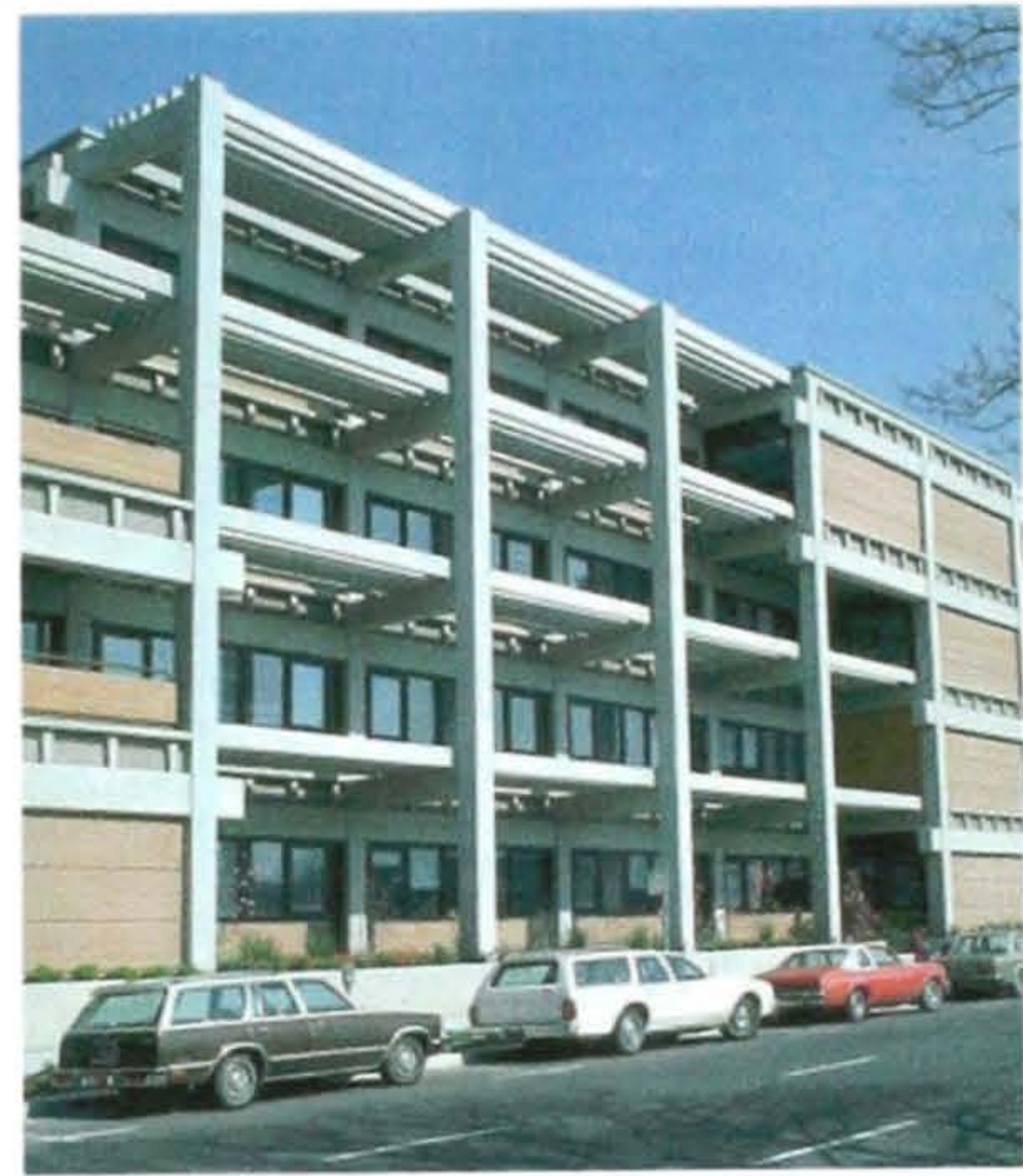
This photo displays the high level of integration employed to both create an inviting appearance and provide shading by emphasizing the concrete structural system.
