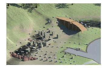
The dam is constructed using stacked lumber that uses dunnage to hold post that run through the dam structure in place. The foundations for the wooden structure are laid as well as masonry walls which will hold the shafts of the sawmill mechanical system.
